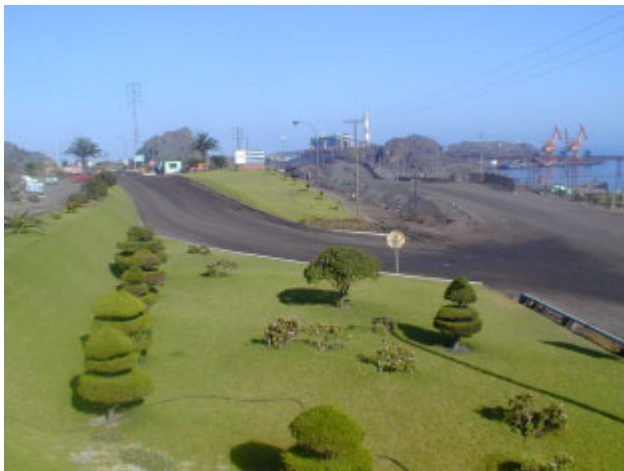
Pellets Plant Main access, Huasco
