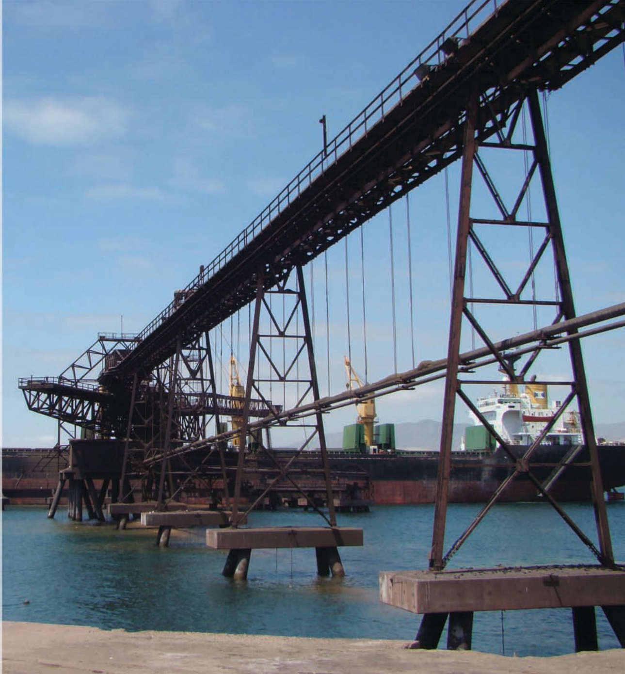
Puerto Guacolda II, Huasco
